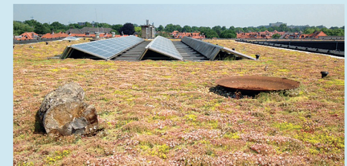
Sedumdak in mei 2018. (Foto: Universal Greenfields)
